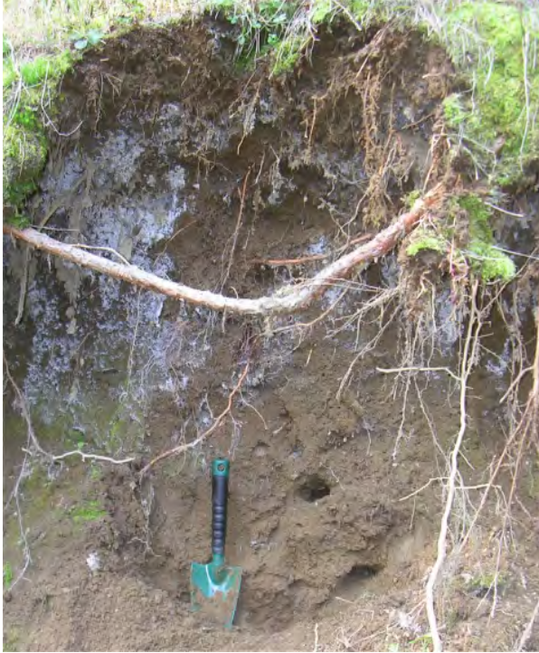
Fig. 5.2.3-1: Typical, abundant colluvial siliceous brown soil of loose sediments with explicit colluvial influence shown in a soil profile and starting point of a landslide in the test area
