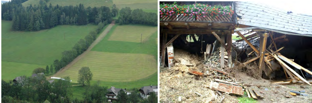
Fig. 3.2-2: The small source area and very long transition and accumulation area of a soil/debris flow (left) and the resulting damage/disaster (right). Photo source: village government photo archives
