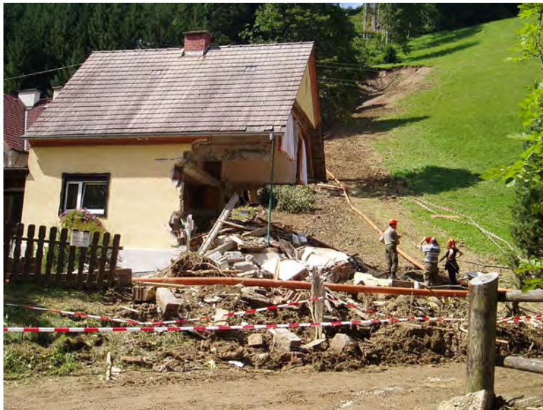
Fig. 3-1: An earth flow/soil flow completely destroyed a home in the village of Gasen. Photo source: GBA photo archives
